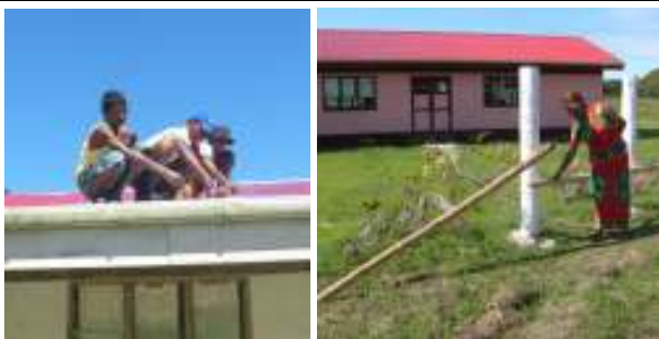
Grade 7 students paint the roof. Teacher and completed wire fence.
